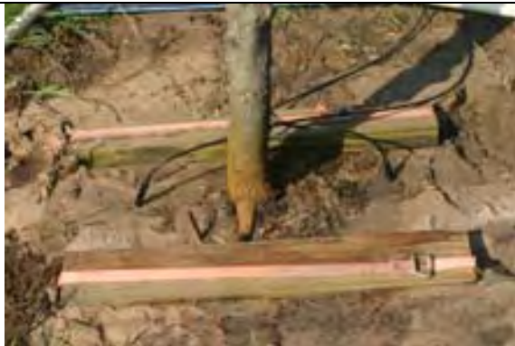
The root ball anchoring system Terra Toggle worked well.
